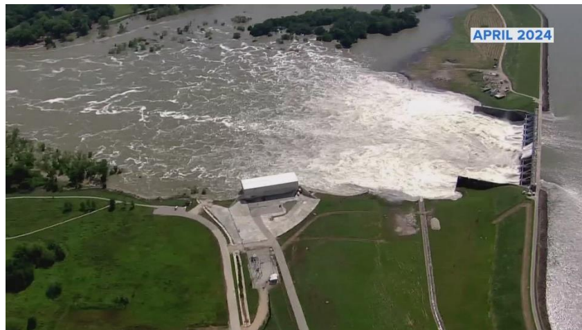
Figure 15-1 Lake Livingston Dam
